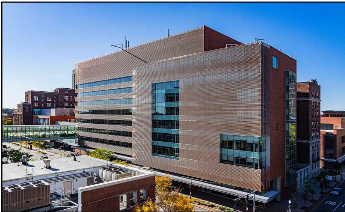
FIGURE 2: In 2012, BMC launched a $350 million campus modernization project that involved renovating 500,000 square feet of existing hospital space and building 130,000 square feet of new clinical space.
