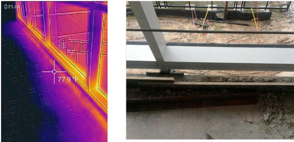
*Figure 3 – Images of curtain wall gap and thermal imagery of gap.*
